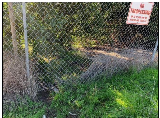
Figure 107. A hole in the fence, animal run, and a No Trespassing sign nearby.
